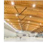
Engineering - Long-Span Structures|StructureCraft
