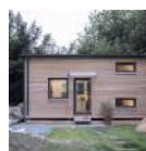
VEKA Windows in Tiny House Village|VEKA
