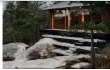
Line Solgaard tops weekend home in Norway with pyramid skylight
